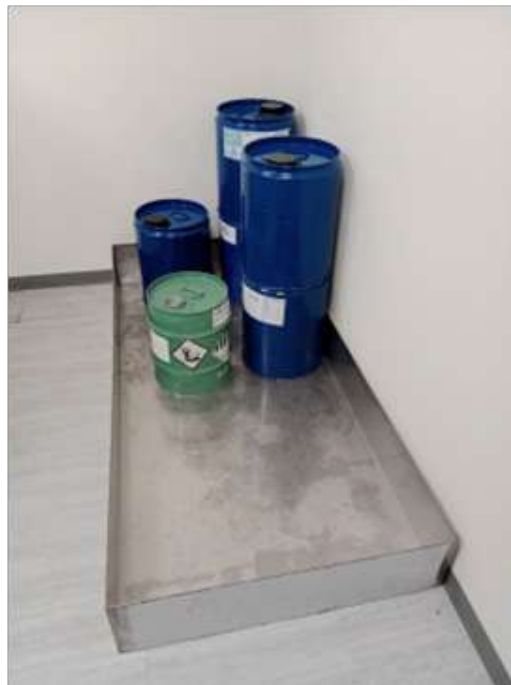
Photo: Large and small spill containment trays at the storage location of organic solvent chemicals
